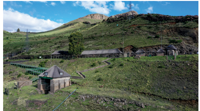
Existing Structure, Mohale Dam.
